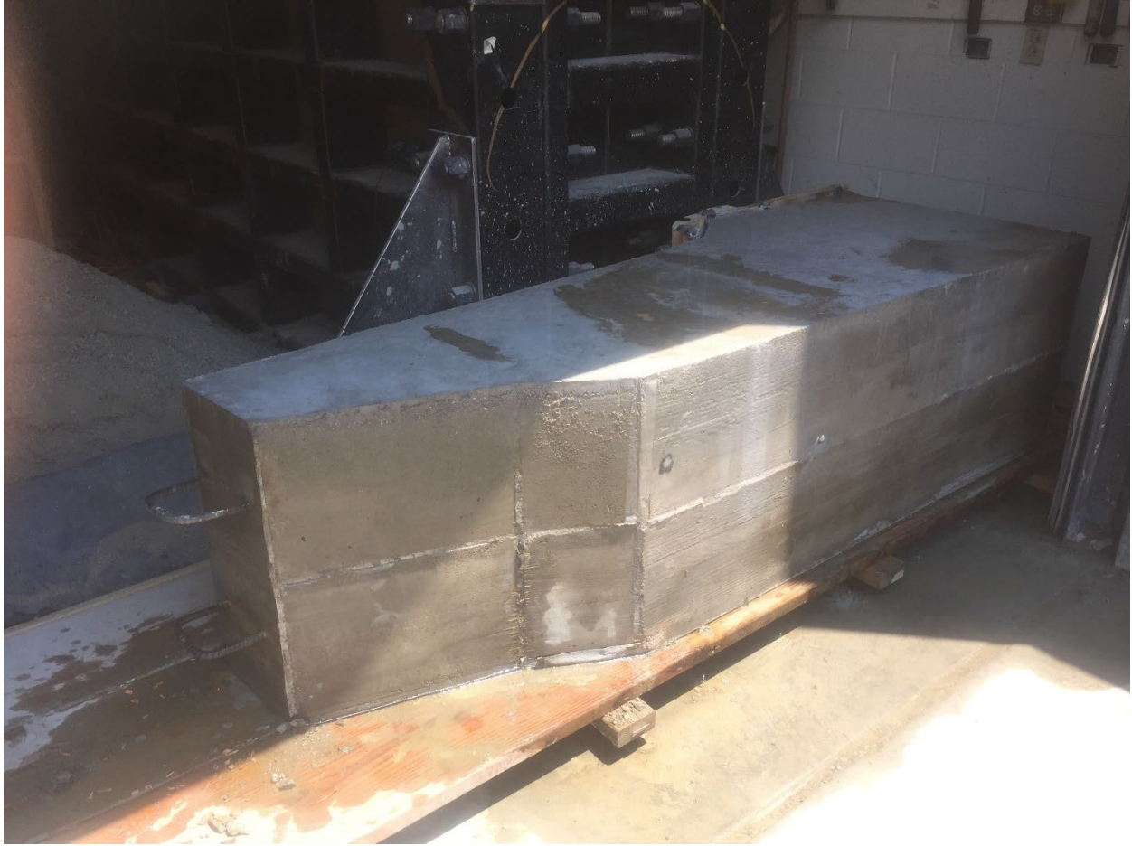
Figure 31. Concrete wall after casting
