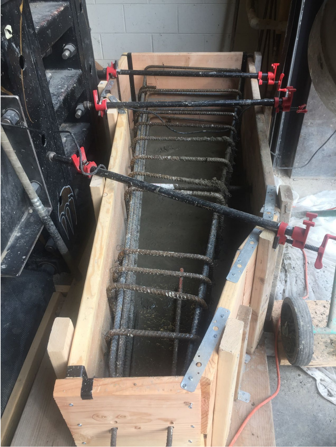
Figure 30. Formwork and reinforcement of the concrete wall
