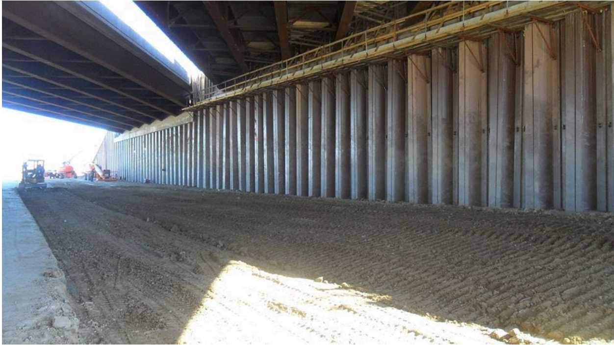
Figure 9. Facing wall of the GRS Abutment #4 (Chang et al., 2020a)
